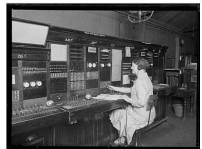
Woman working the London switchboard at the General Post Office in Sydney, New South Wales, 24 March 1932 [picture]. Source: National Library of Australia
