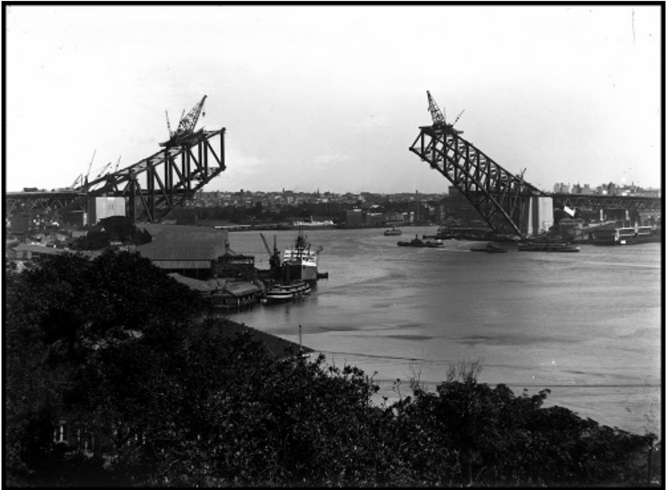
Both sides of Sydney Harbour Bridge from North Sydney, 5 panels on north. Photographed by Frank Cash.
